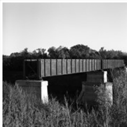
Abandoned bridge over Souris River at Wawanesa, Manitoba
