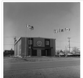
Dakota-Ojibway Tribal Council Building
