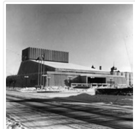
Western Manitoba Centennial Auditorium
