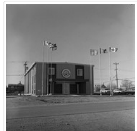
Dakota-Ojibway Tribal Council Building
