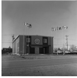
Dakota-Ojibway Tribal Council Building
