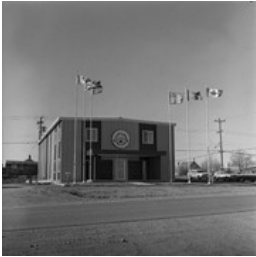
Dakota-Ojibway Tribal Council Building
