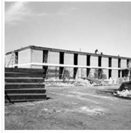
Brandon College - building construction
