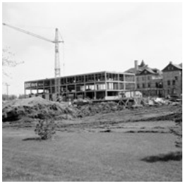
Brandon College - building construction
