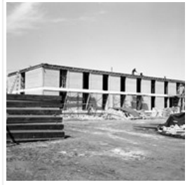
Brandon College - building construction
