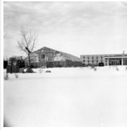
Brandon College - building construction
