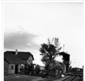
CP 5233, station, water tank, and elevator. Binscarth, ...
