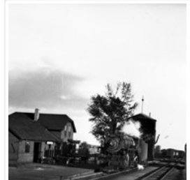
CP 5233, station, water tank, and elevator. Binscarth, ...
