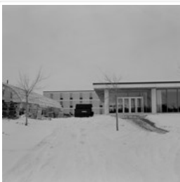
Brandon College - building construction
