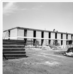
Brandon College - building construction
