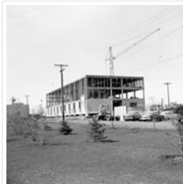
Brandon College - building construction
