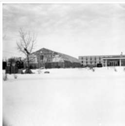
Brandon College - building construction
