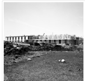
Brandon College - building construction
