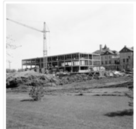
Brandon College - building construction
