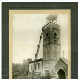
Original Fire Hall
