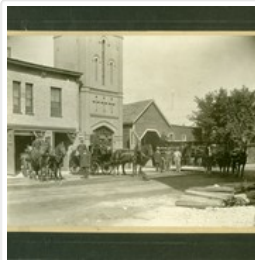
Original Fire Hall
