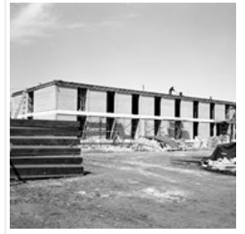
Brandon College - building construction
