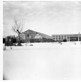
Brandon College - building construction
