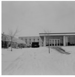
Brandon College - building construction
