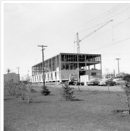
Brandon College - building construction
