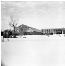
Brandon College - building construction
