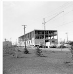
Brandon College - building construction
