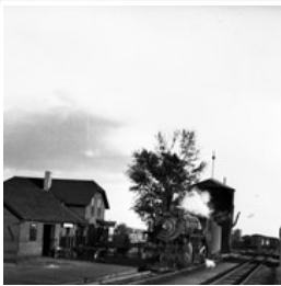
CP 5233, station, water tank, and elevator. Binscarth, ...
