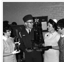
Air Force inspection
