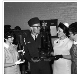
Air Force inspection
