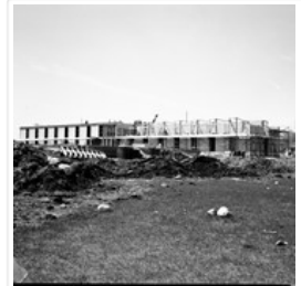
Brandon College - building construction
