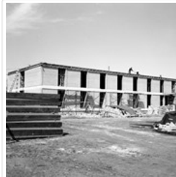
Brandon College - building construction
