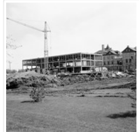
Brandon College - building construction
