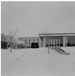
Brandon College - building construction
