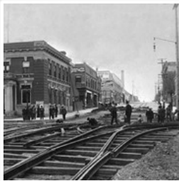
Brandon Municipal Railway Construction
