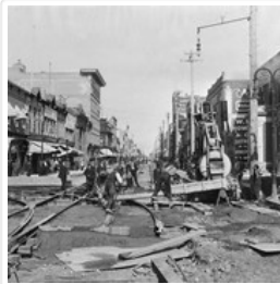
Brandon Municipal Railway Construction
