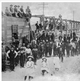
Sewer Line Construction
