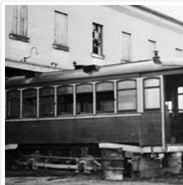
Dismantling of Streetcar No. 8
