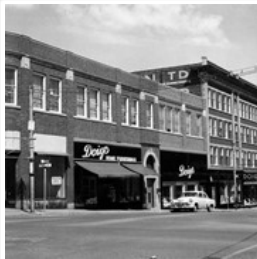
10th Street Businesses - West Side of 100 ...
