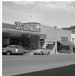
10th Street Businesses - West Side of 100 ...
