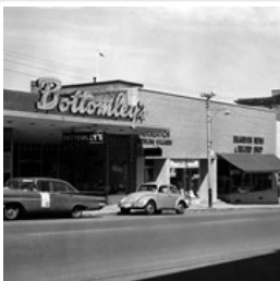
10th Street Businesses - West Side of 100 ...
