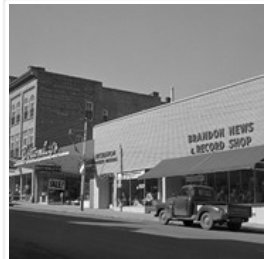
10th Street Businesses - West Side of 100 ...
