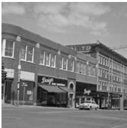
10th Street Businesses - West Side of 100 ...
