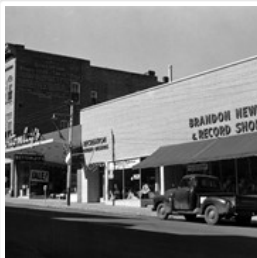
10th Street Businesses - West Side of 100 ...
