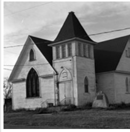
Former Church, now Community Hall, Chater, Manitoba.
