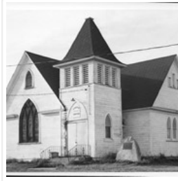
Former Church, now Community Hall, Chater, Manitoba.
