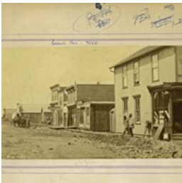
Rosser Avenue, north side 900 block
