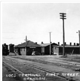
CNR Engine Terminal
