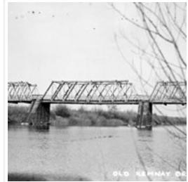
Assiniboine River Bridge North of Kemnay
