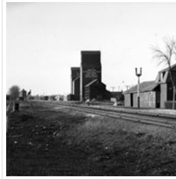
CPR Station and Lineside buildings, Reston, Manitoba
