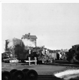
CNR Engine Terminal
