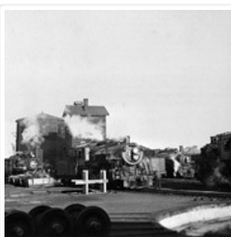
CNR Engine Terminal
