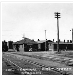
CNR Engine Terminal
