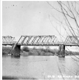
Assiniboine River Bridge North of Kemnay
