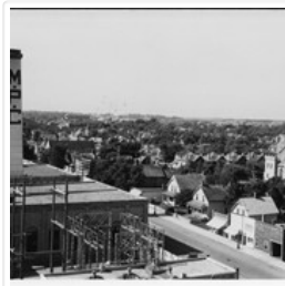
Aerial view of 10th Street facing south from ...
