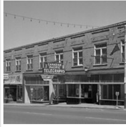
10th Street Commercial Block
