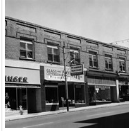
10th Street Commercial Block
