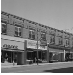
10th Street Commercial Block
