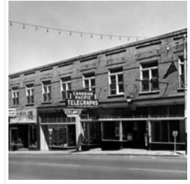
10th Street Commercial Block
