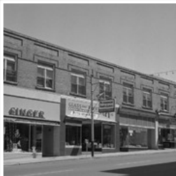
10th Street Commercial Block
