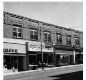
10th Street Commercial Block
