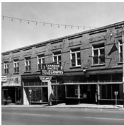
10th Street Commercial Block
