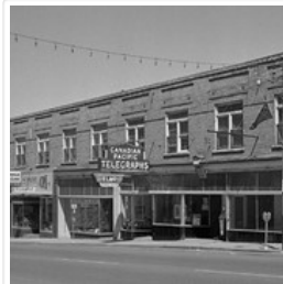
10th Street Commercial Block
