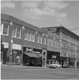
10th Street Businesses - West Side of 100 ...
