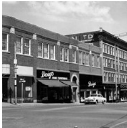
10th Street Businesses - West Side of 100 ...
