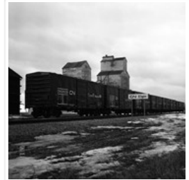
Grain elevators, Elgin, Manitoba
