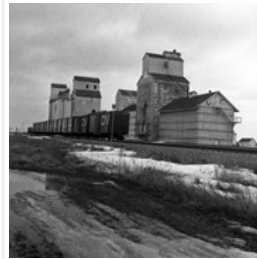
Grain elevators, Elgin, Manitoba
