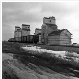
Grain elevators, Elgin, Manitoba
