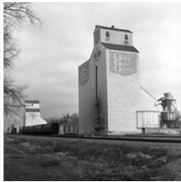
Grain elevators, Hartney, Manitoba
