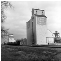
Grain elevators, Hartney, Manitoba
