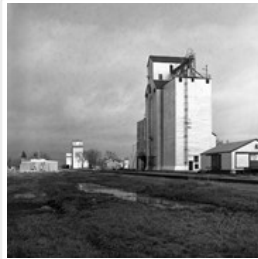
Grain elevators, Hartney, Manitoba
