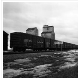
Grain elevators, Elgin, Manitoba
