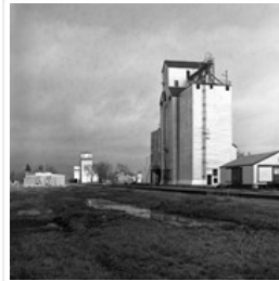
Grain elevators, Hartney, Manitoba
