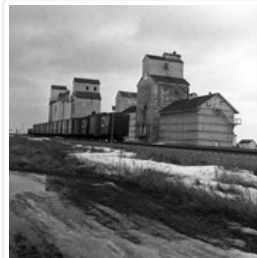
Grain elevators, Elgin, Manitoba
