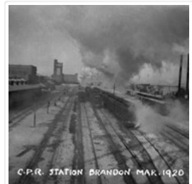
CPR Station and Coach Yard - Showing Heating ...
