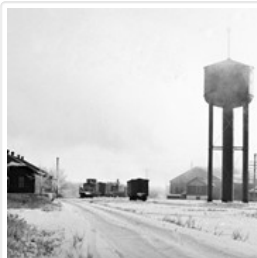
CPR Shop Buildings, Water Tower, and Bunkhouse
