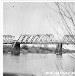
Assiniboine River Bridge North of Kemnay
