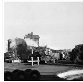
CNR Engine Terminal
