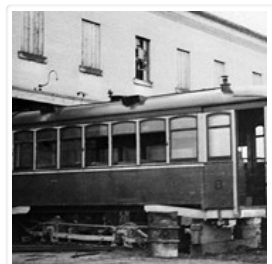
Dismantling of Streetcar No. 8
