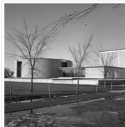
Brandon College - old and new buildings
