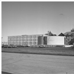
Brandon College - old and new buildings
