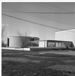
Brandon College - old and new buildings
