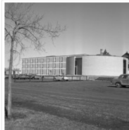
Brandon College - old and new buildings
