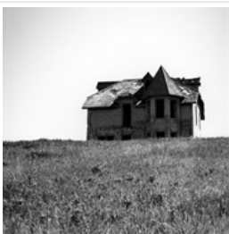
Old concrete house
