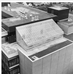
Aerial view: John R. Brodie Science Centre roof ...
