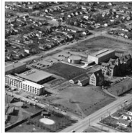
Aerial view: Brandon College Steam Plant
