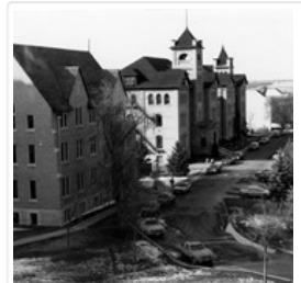
Aerial view: Citizens' Science Building
