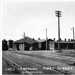
CNR Engine Terminal
