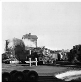
CNR Engine Terminal
