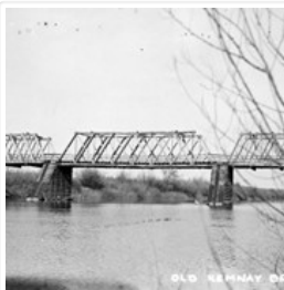
Assiniboine River Bridge North of Kemnay
