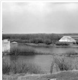
Grand Trunk Pacific Bridge Piers
