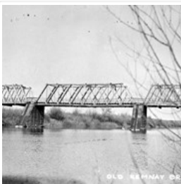
Assiniboine River Bridge North of Kemnay
