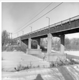
Second First Street bridge
