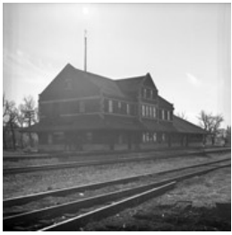
CPR station and engine at sand dock. Souris, ...
