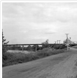
Construction of third First Street bridge
