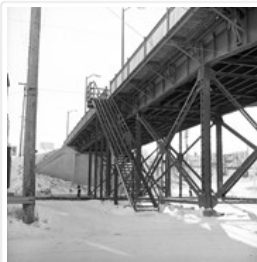
Second First Street bridge
