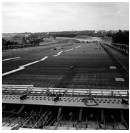
Construction of third First Street bridge
