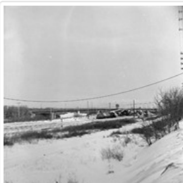
Second First Street bridge
