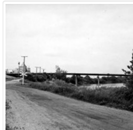
Construction of third First Street bridge
