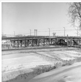
Second First Street bridge
