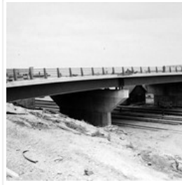
Construction of third First Street bridge
