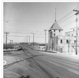
Second First Street bridge
