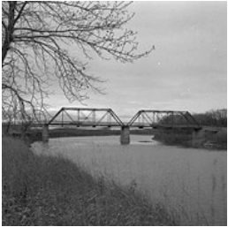
Second 18th Street bridge
