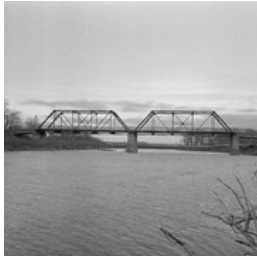
Second 18th Street bridge
