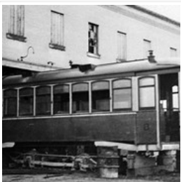
Dismantling of Streetcar No. 8
