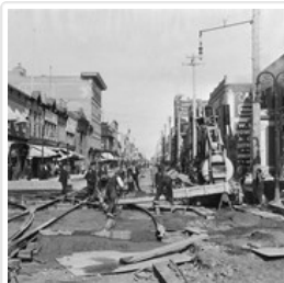
Brandon Municipal Railway Construction
