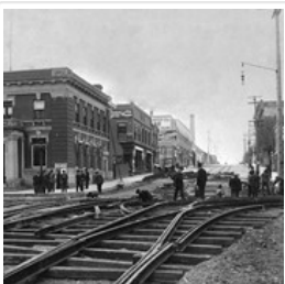
Brandon Municipal Railway Construction
