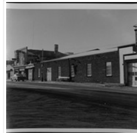
West side 200-block 10th Street facing south from ...
