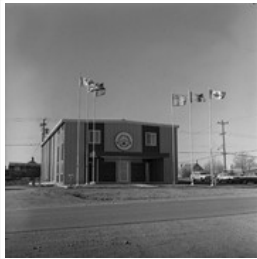
Dakota-Ojibway Tribal Council Building
