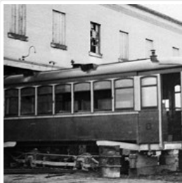
Dismantling of Streetcar No. 8
