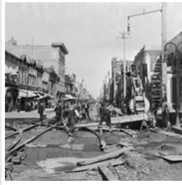
Brandon Municipal Railway Construction
