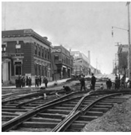
Brandon Municipal Railway Construction
