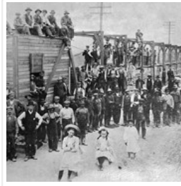
Sewer Line Construction
