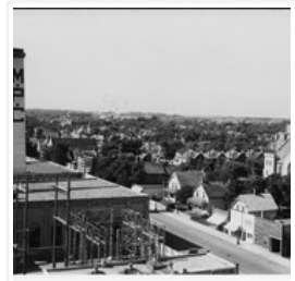
Aerial view of 10th Street facing south from ...
