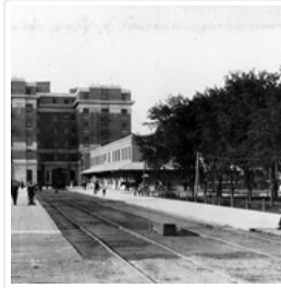
Canadian Northern Railway depot
