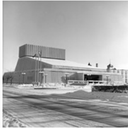
Western Manitoba Centennial Auditorium
