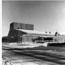
Western Manitoba Centennial Auditorium
