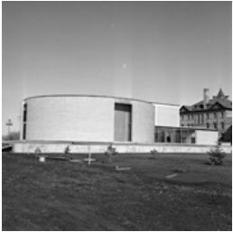
Brandon College - old and new buildings
