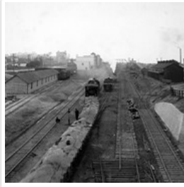
Canadian Pacific Railway tracks from 1st street bridge ...
