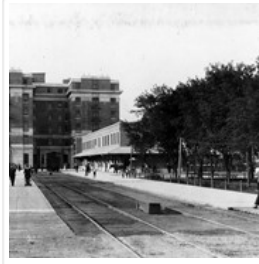
Canadian Northern Railway depot
