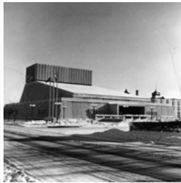
Western Manitoba Centennial Auditorium
