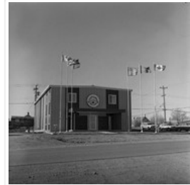
Dakota-Ojibway Tribal Council Building
