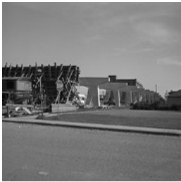
Eighteenth Street Overpass Construction
